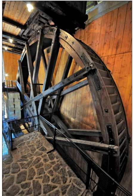
The wooden water wheel of the Idrija Kamšt water pump.
