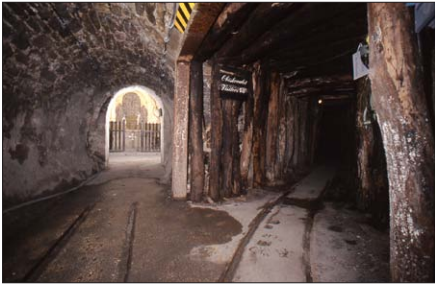
Main galleries with the underground Chapel of the Holy Trinity still open to the public, Idrija.
